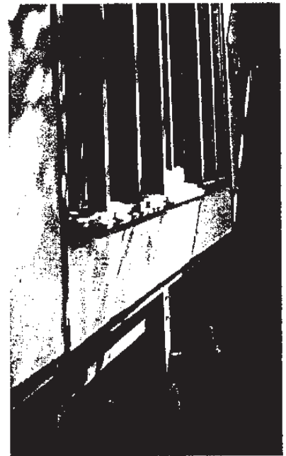
Figure 61: Post ends resting on concrete piers precast in a bucket, at the Centre for Alternative Technology, Mid-Wales.
