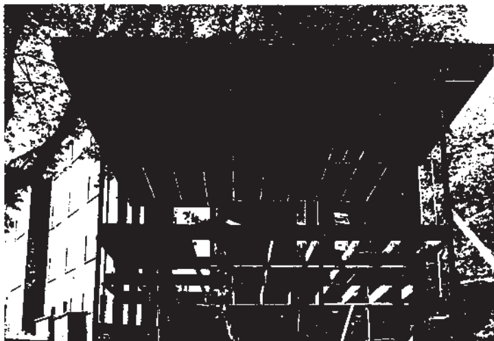
Figure 63: Flat roof frames on the Lewisham self build house (1980)
