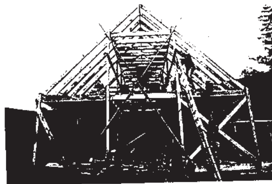
Figure 66: Three-bay purlin framed house at C.A.T.
